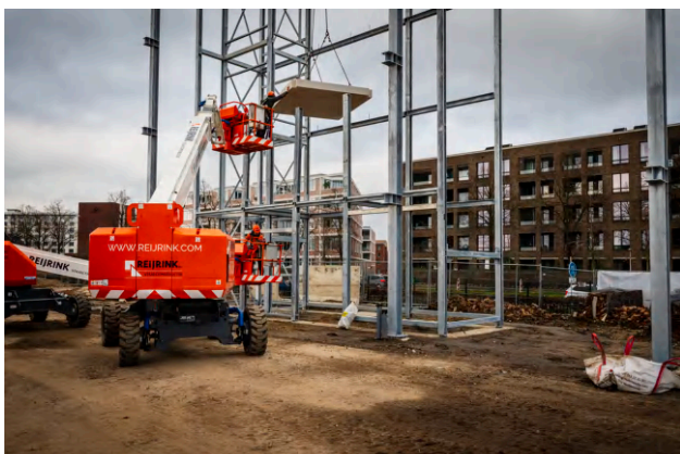
Figure 5: Assembling the prefabricated elements
