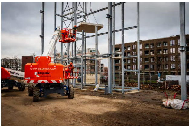
Figure 5: Assembling the prefabricated elements
